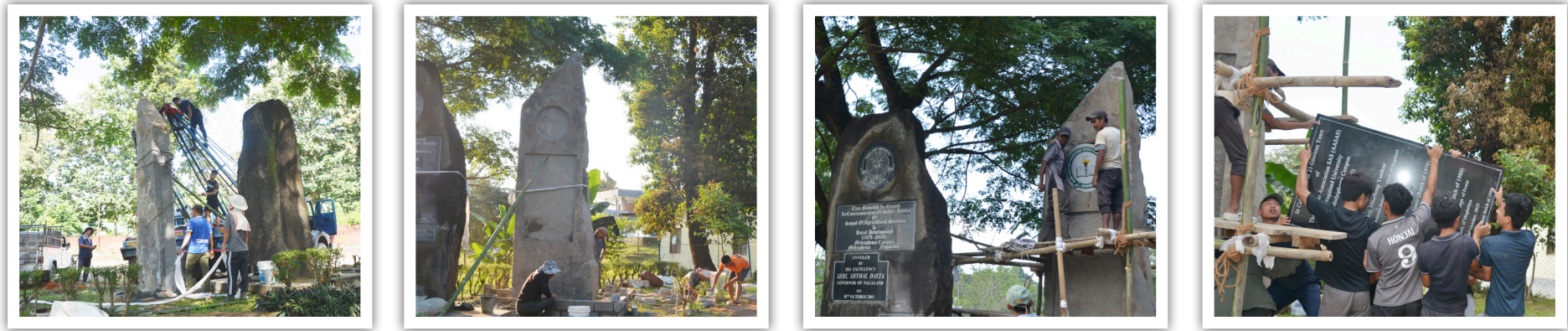
In preparation of Monolith Installation
